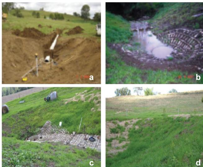
Figure 6. (a) Installing the concrete pipe, (b) Flood waters leaving the stilling basin, (c) The reshaped gully head area, (d) The end result; mostly grass to look at.
