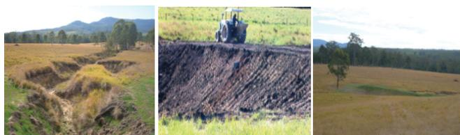
**Figure 8.** (a) Looking down the gully (b) Spreading seed and fertiliser (c) The finished dam
